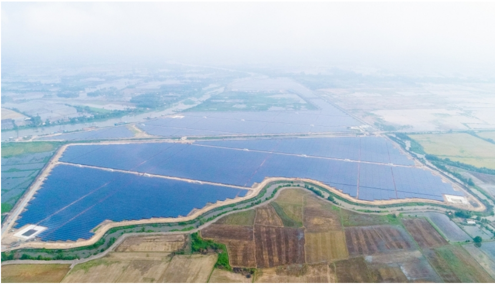
TTC No.01 and No.02 solar power plants in Thanh Thanh Cong Industrial Zone, Tay Ninh province
